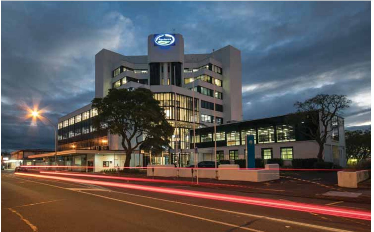
Fonterra House, Hamilton (Wholly owned investment property in New Zealand)
